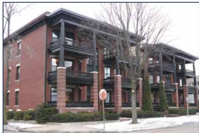
Example of multi-family housing with downtown character.
