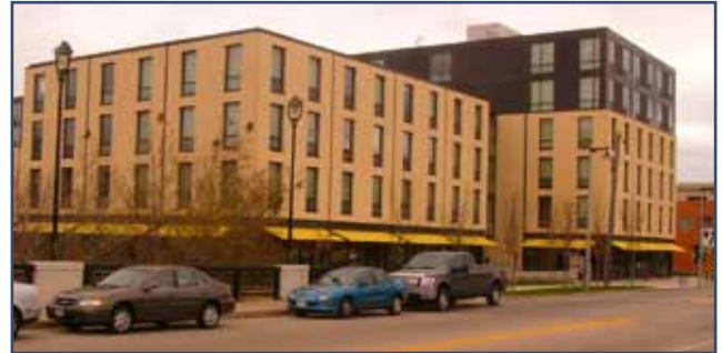
Recently completed UW-Milwaukee off-campus housing with retail along the ground level
