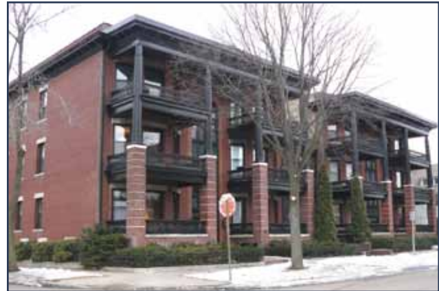
Example of multi-family housing with downtown character.
