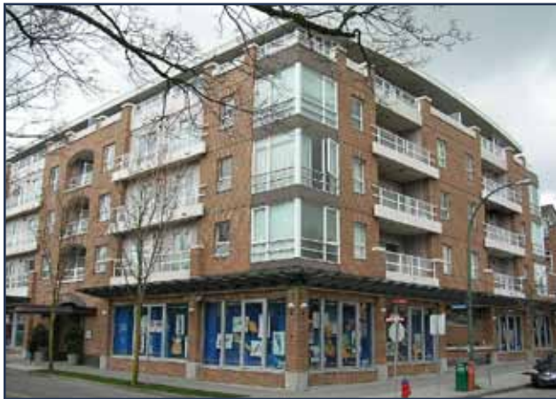
Example of mixed-development with the top story set back from the primary facade.
