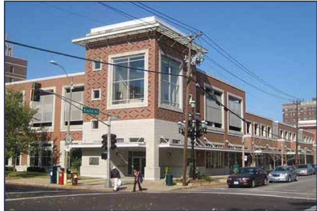
Example of two-story parking ramp.
