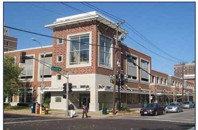
Example of two-story parking ramp.
