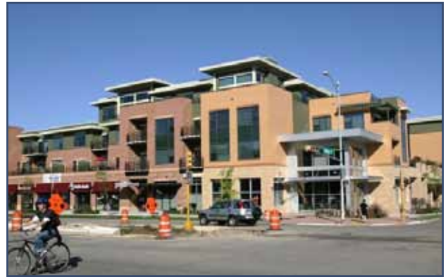
Example of mixed-use development with retail, residential, and a library center.
