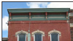
FLAT ROOF W/ CORNICE
