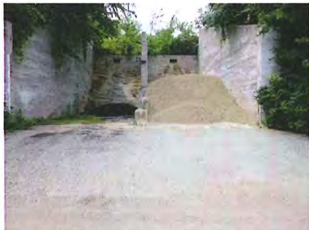
Figure 17: Water Plant Uncovered Stockpiles
