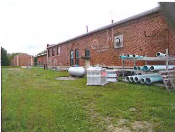
Figure 16: Water Plant Outdoor Storage
