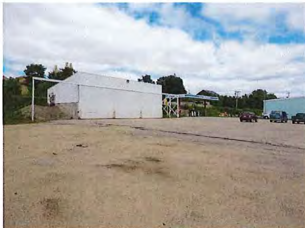
Figure 13: Salt Storage Shed and Fueling Tanks
