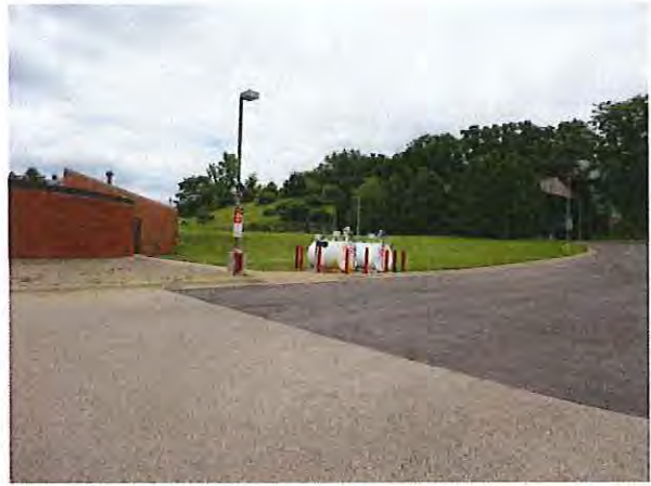
Figure 6: WWTF Fuel Tanks
