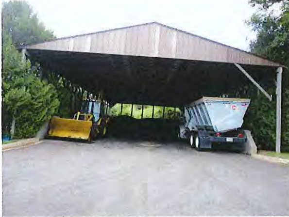
Figure 5: WWTF Sludge Storage Shed
