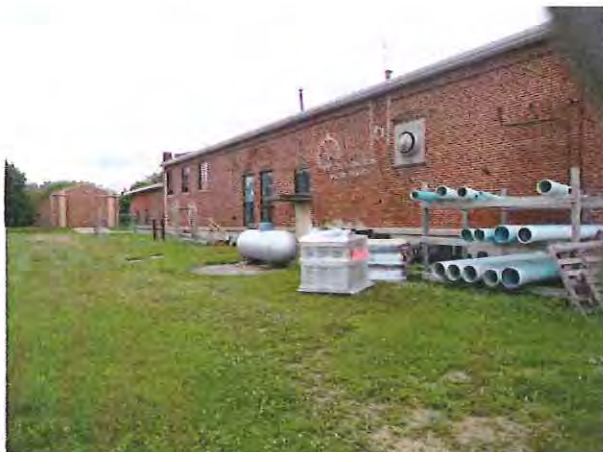
Figure 16: Water Plant Outdoor Storage
