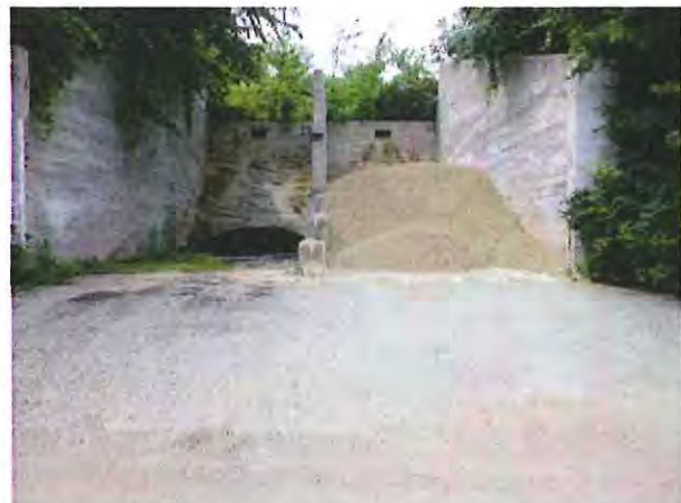
Figure 17: Water Plant Uncovered Stockpiles
