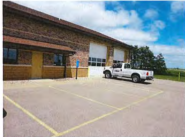
Figure 20: Municipal Well #5, Garage, and Office
