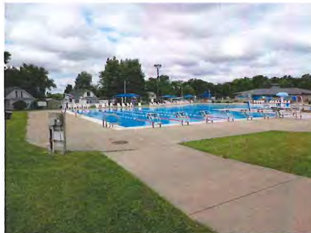
Figure 10: Platteville Family Aquatic Center
