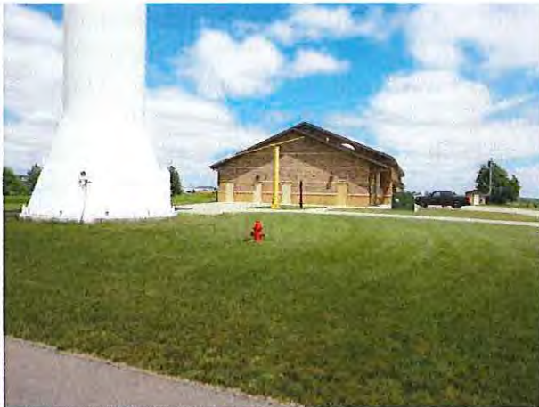
Figure 19: Industry Park Water Tower
