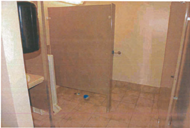
Lower Level Restroom
