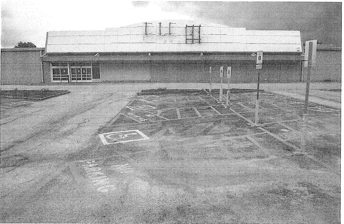
The shuttered Kmart store in Rock Island sits vacant on Monday Aug. 15, 2016.
