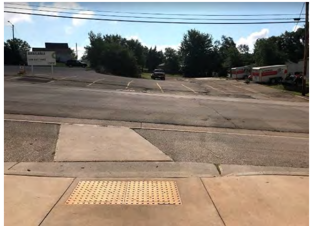
Figure 1 Location for mid-block crossing
