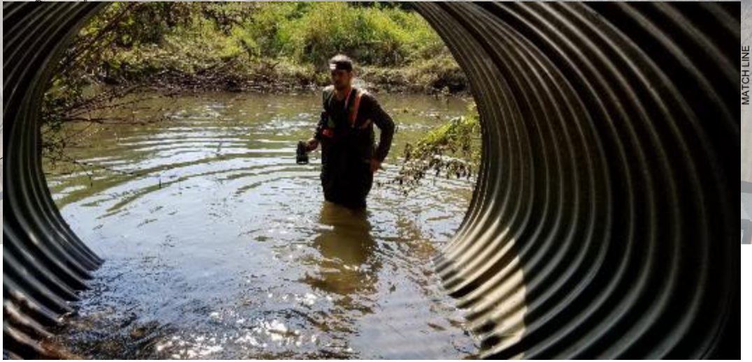
Discharge is submerged and no endwall
