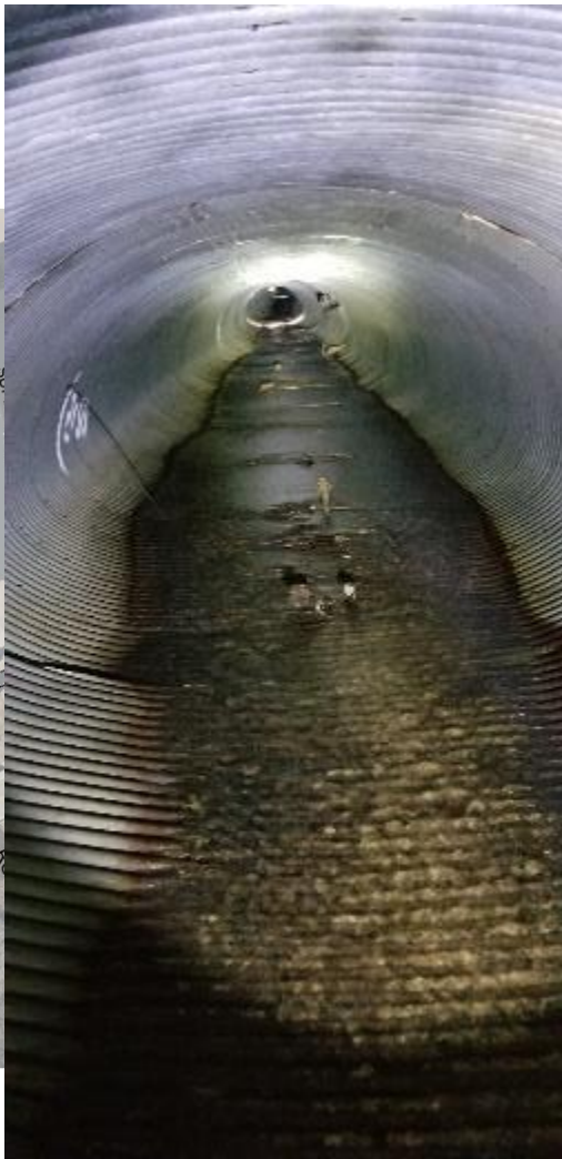
Bottom of CMP culvert has rusted through
