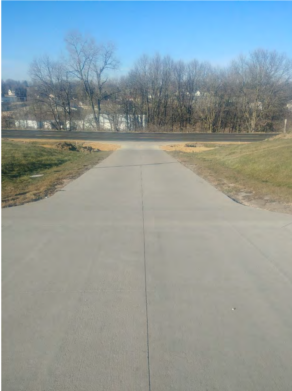
Driveway viewing north toward Bus 151
