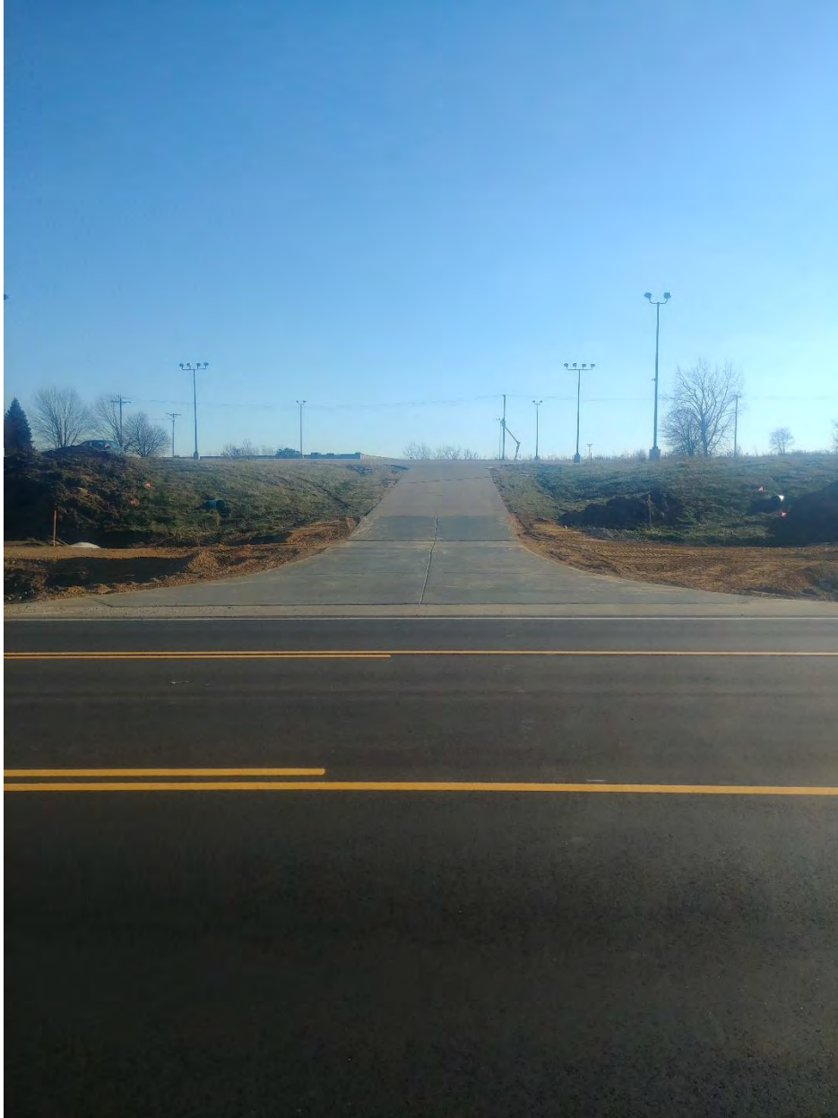
Driveway viewing south from Bus 151
