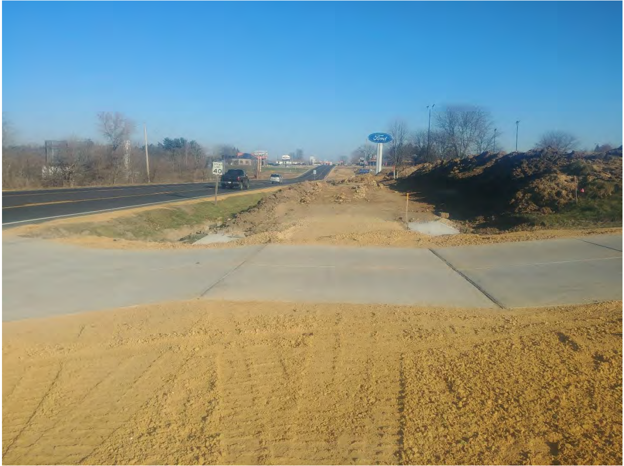
Trail crossing driveway viewing east
