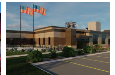
Kenosha Station 4: 29,344 s.f. - $9,260,000 scheduled to be delivered ahead of schedule and under budget
