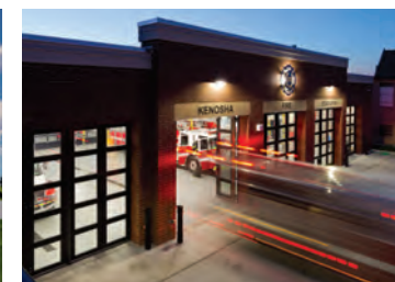
Kenosha Station 1: 23,895 s.f. - $5,250,000 delivered one month ahead of schedule and under budget
