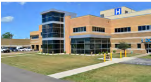
CAMPUS CLINIC ADDITION - 2013
