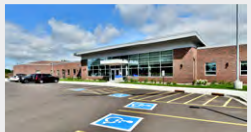
CVTC FIRE TRAINING CENTER
