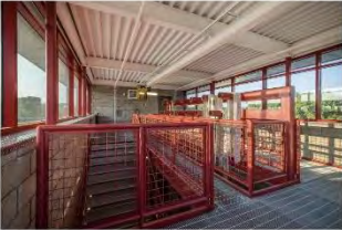
UPPER PLATFORM: HOSE DRYING, STANDPIPE, ROOF ACCESS
