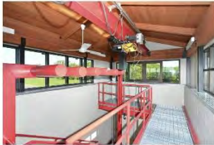
UPPER PLATFORM: HOSE DRYING, INTERIOR RAPPILING, STANDPIPE, OPERABLE TRAINING WINDOW
