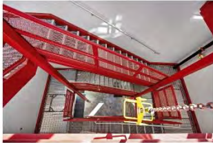
OVERALL VIEW OF TRAINING TOWER STAIR FROM ABOVE
