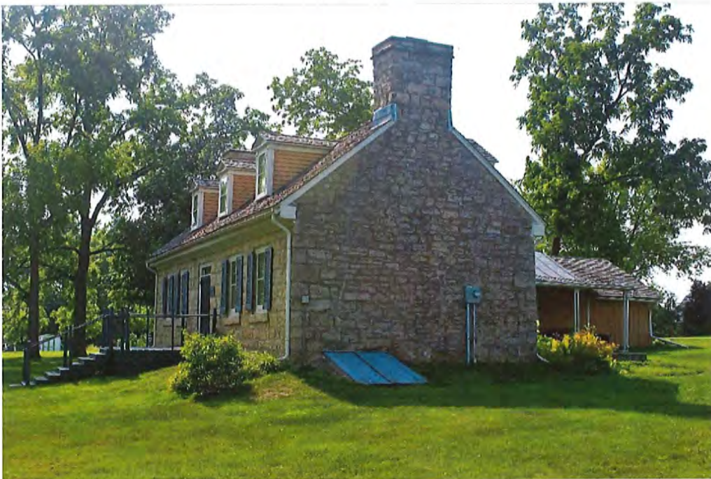
Side view, (East, southeast facing)
