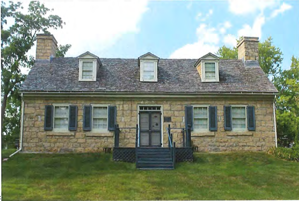
Front view (South facing)
