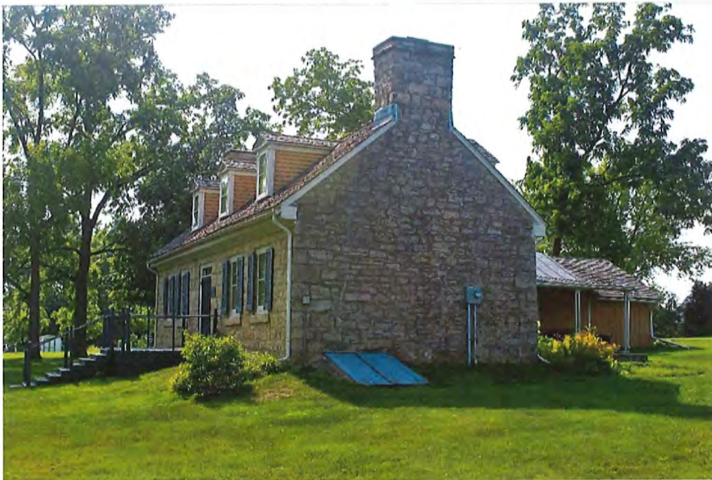
Side view, (East, southeast facing)
