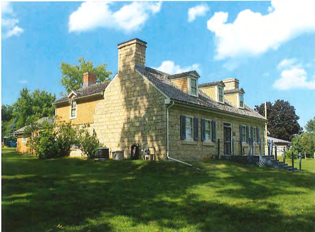
West, southwest view
