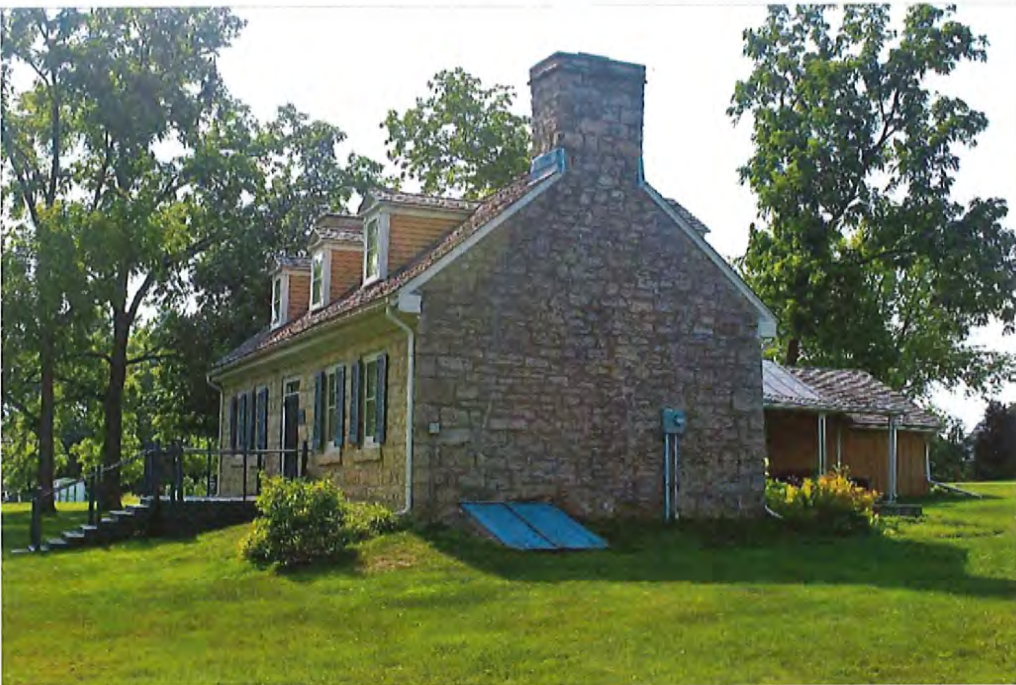
Side view, (East, southeast facing)
