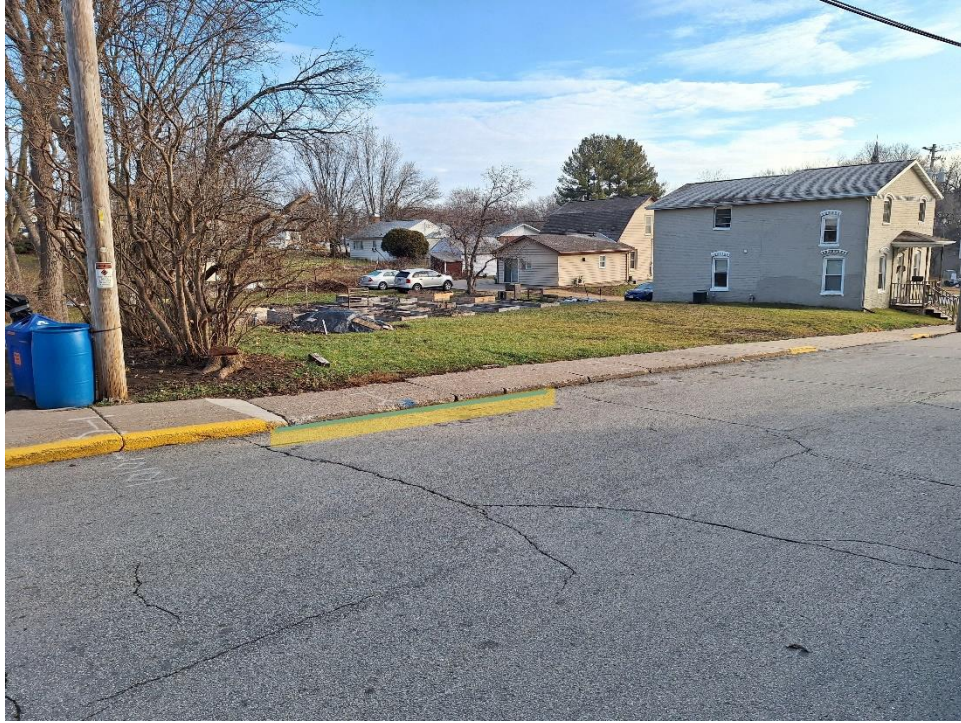
North side parking space to be eliminated – note the hand drawn yellow
