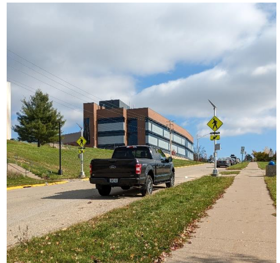
Figure 3: RRFB at Southwest Road and UWP Lot 28
