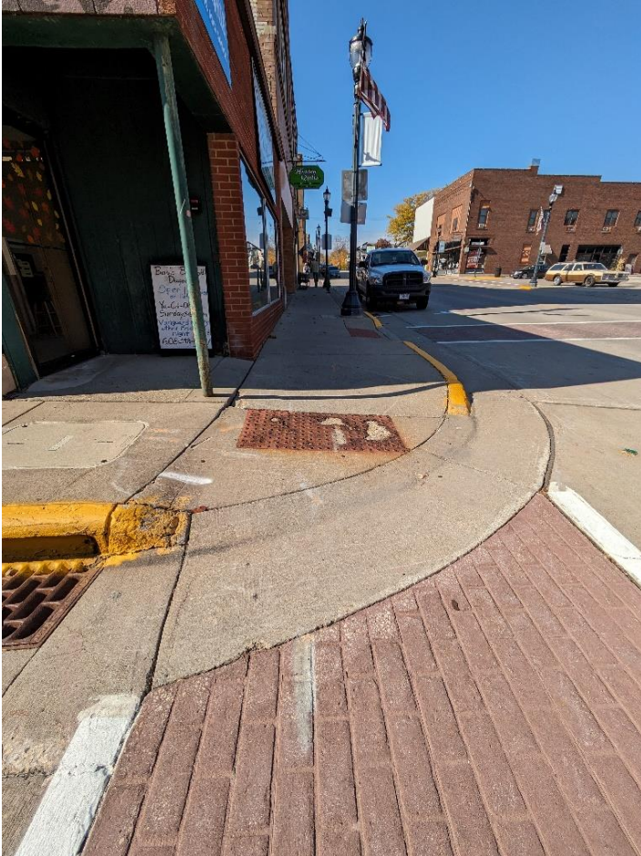
Figure 27: Broken ADA ramp (left, SW corner of Main and Bonson) and noncompliant ramp (right, SW corner of Southwest and Hickory)
