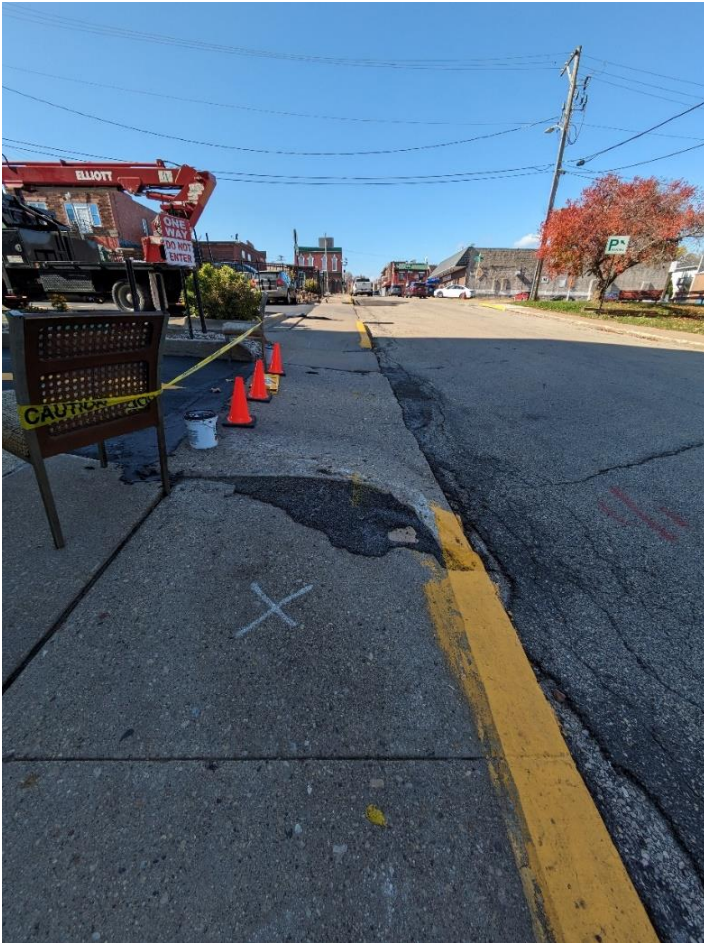
Figure 21: Cracks and uneven sidewalk on the south side of Mineral Street near Jenor Towers
