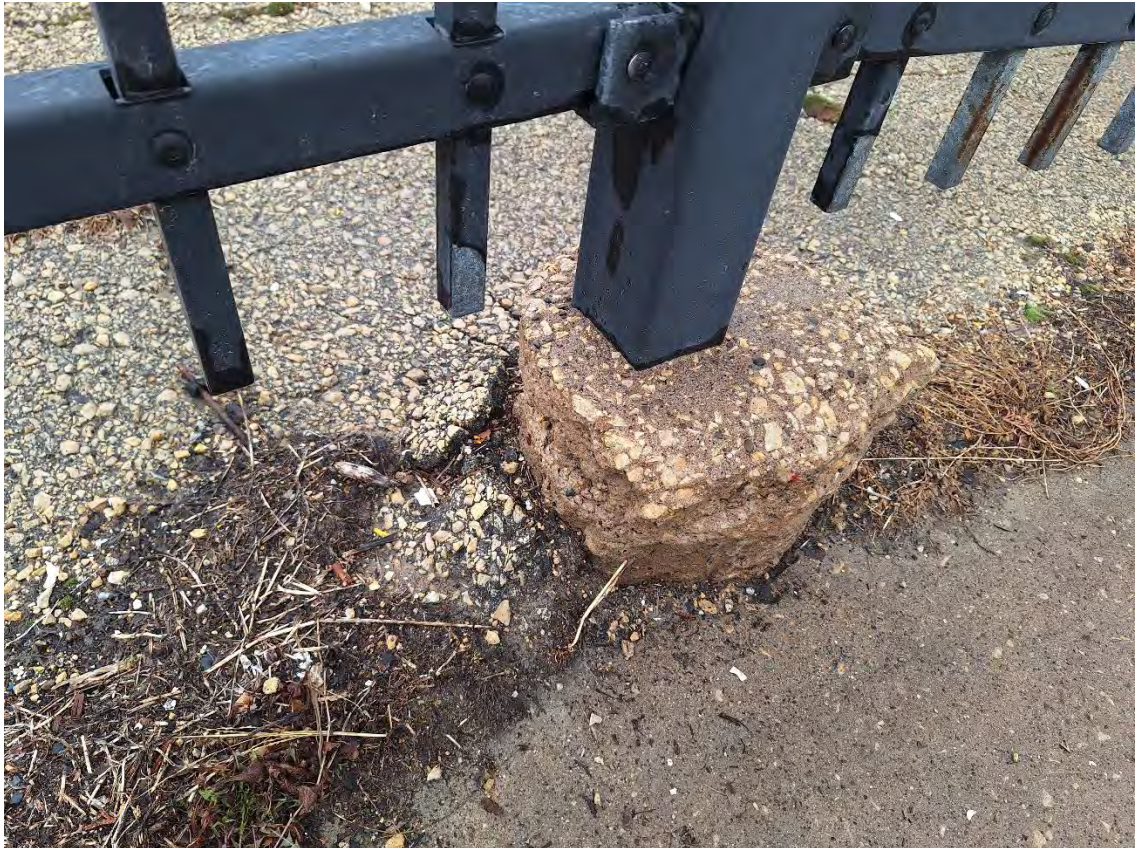
Fencepost anchored in concrete. Concrete heaved over the years. Unknown cost to carefully remove the posts and knock off the old concrete.
