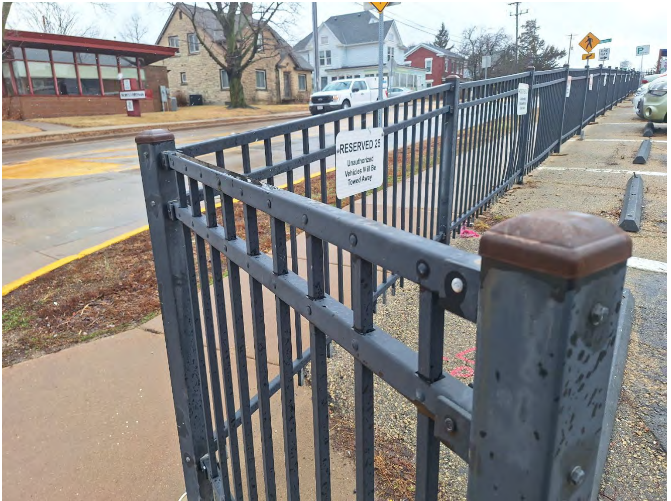
Rusted Fence caps. All are in similar condition. Unknown cost to sandblast and re-paint.
