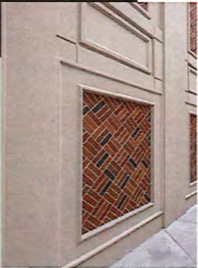
ILLS, COPINGS & FASCIES - ACID ETCHED PRECAST
