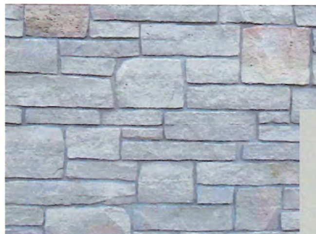
EXTERIOR STONE MASONRY - FOND DU LAC STONE - "HAMILTON COUNTRY" LARGE FORMAT STONE IS THE SAME STONE, JUST CUT LARGER
