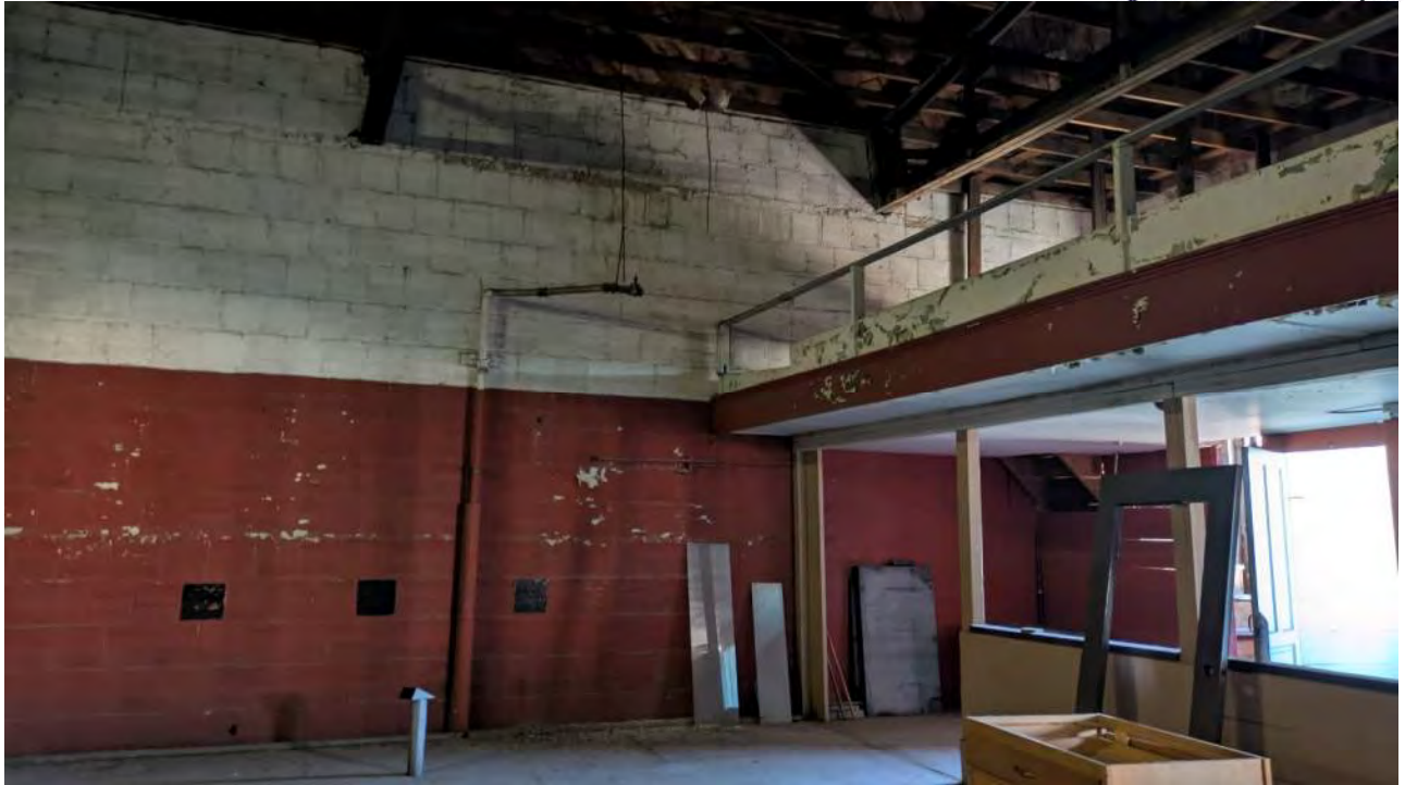
Photo 3 – East wall, Upper Level showing clay tile wall and truss bearing
