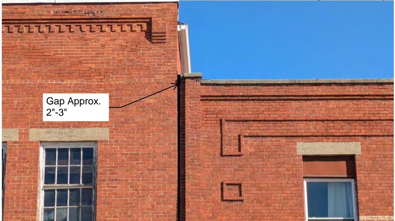
Photo 13 – Exterior, Joint between 230 & 250 E Main Street
