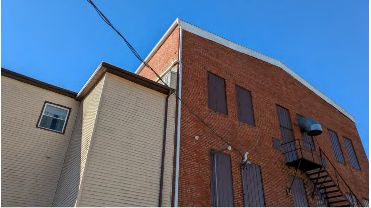
Photo 21 – Joint between buildings on North wall
