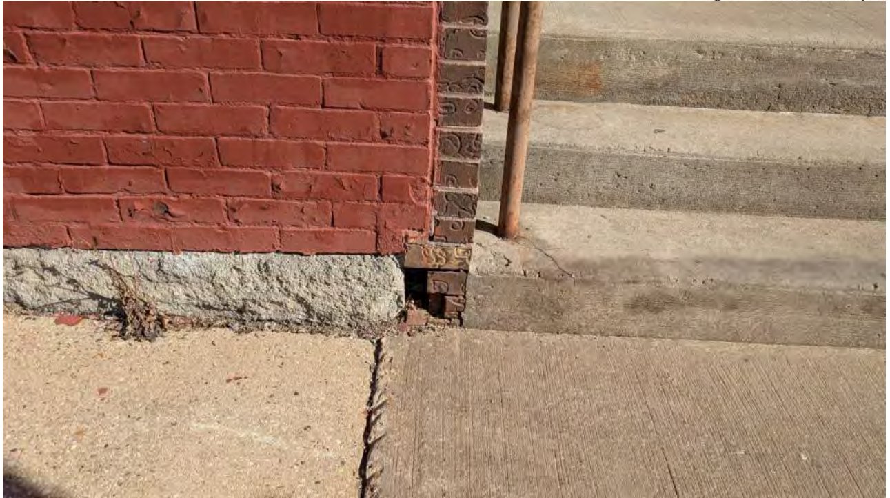
Photo 17 – Exterior, Joint between 230 & 250 E Main Street
