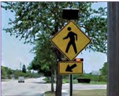
Figure 2: Activated, solar-powered, roadside RRFB at a mid-block crosswalk
