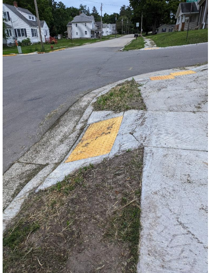
Figure 27: Broken ADA ramp (left, SW corner of Main and Bonson) and noncompliant ramp (right, SW corner of Southwest and Hickory)
