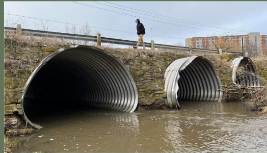
Figure 3: Existing Masonry Wall, Looking Northeast
