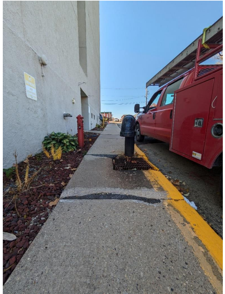
Figure 21: Cracks and uneven sidewalk on the south side of Mineral Street near Jenor Towers
