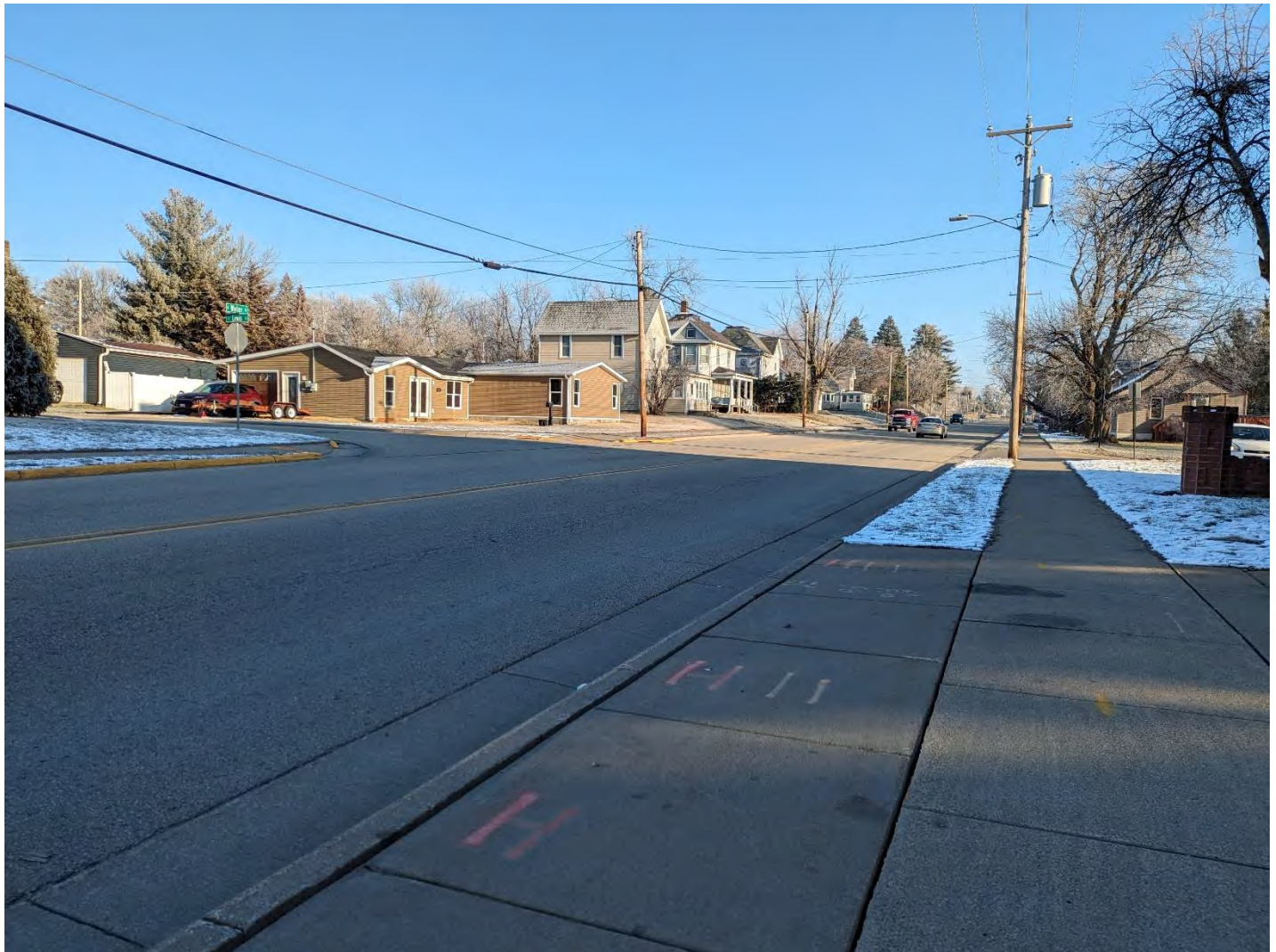
Figure 20: Intersection of Water Street and Lewis Street with the Armory to the right
