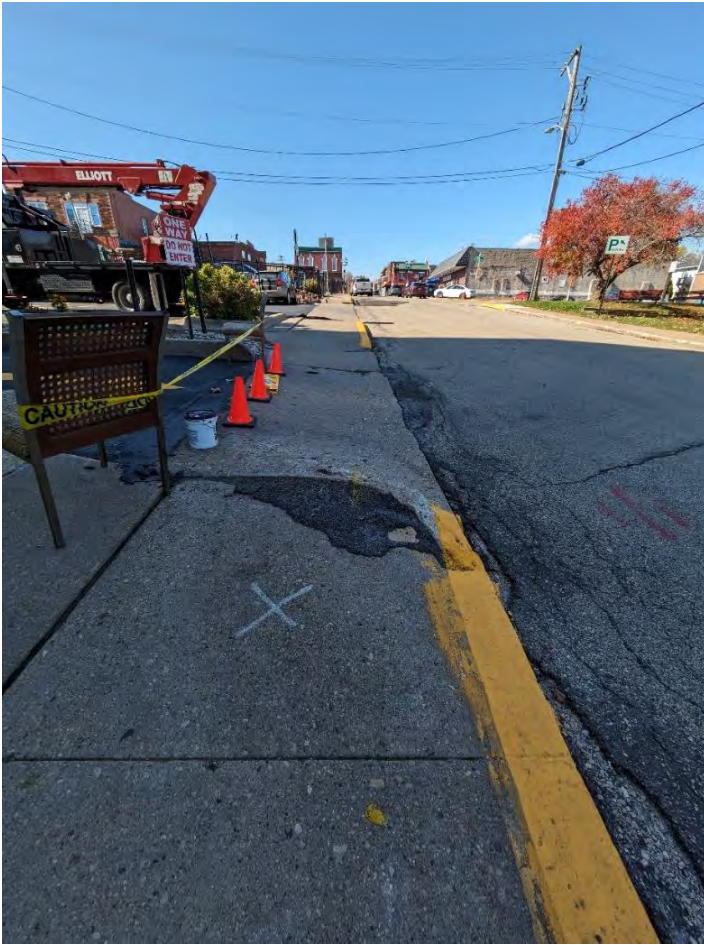
Figure 19: Cracks and uneven sidewalk on the south side of Mineral Street near Jenor Towers
