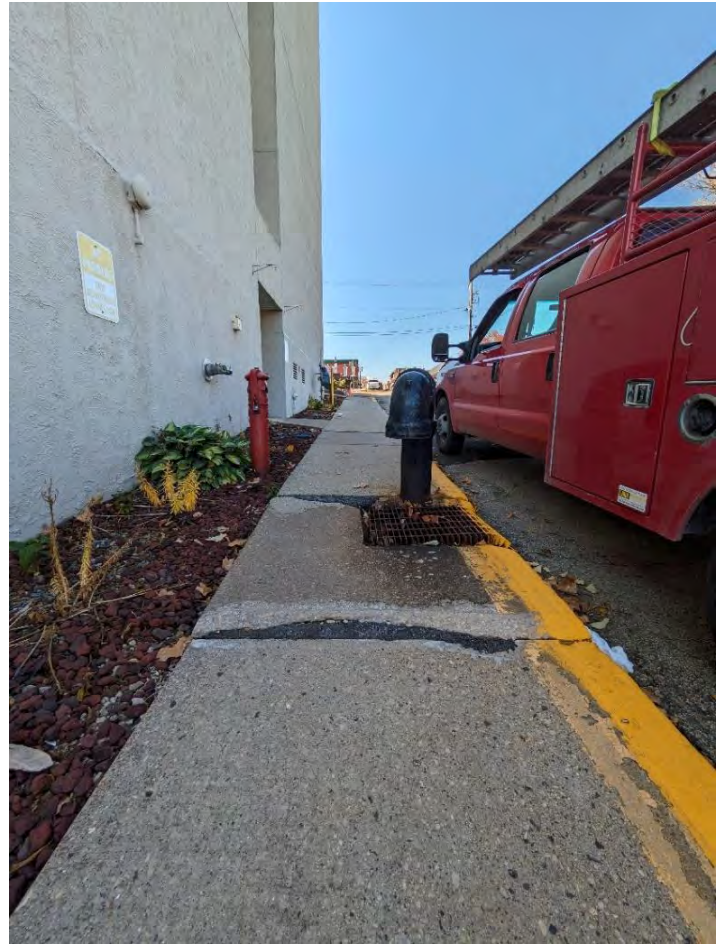
Figure 19: Cracks and uneven sidewalk on the south side of Mineral Street near Jenor Towers
