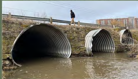
Figure 3: Existing Masonry Wall, Looking Northeast
