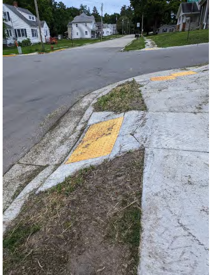
Figure 25: Broken ADA ramp (left, SW corner of Main and Bonson) and noncompliant ramp (right, SW corner of Southwest and Hickory)
