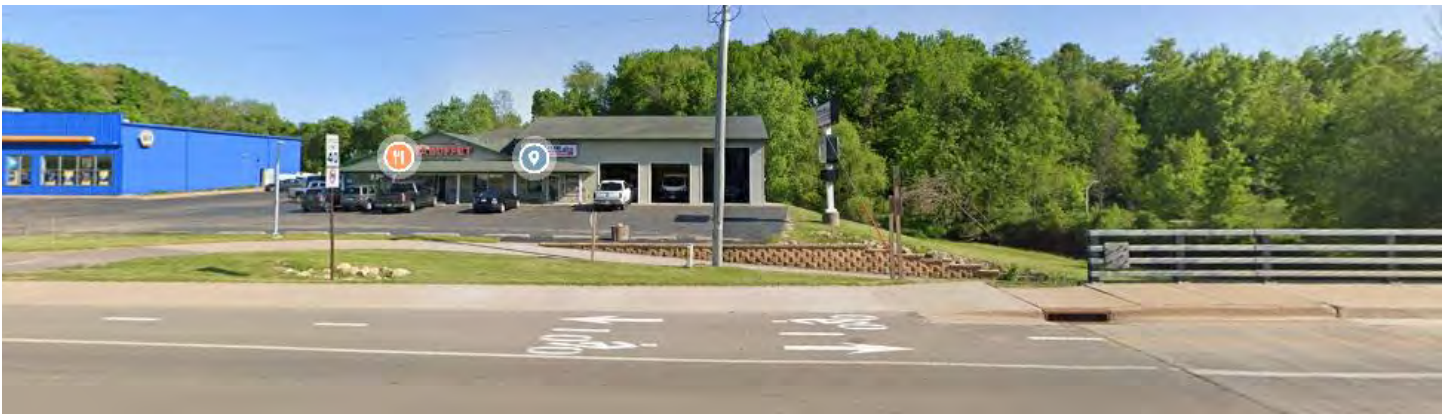
Figure 35: Bike lane and raised sidewalk on Business 151 bridge 18
