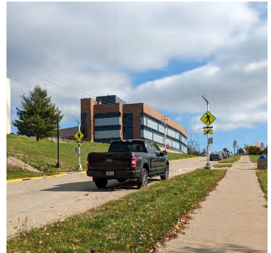
Figure 3: RRFB at Southwest Road and UWP Lot 28
