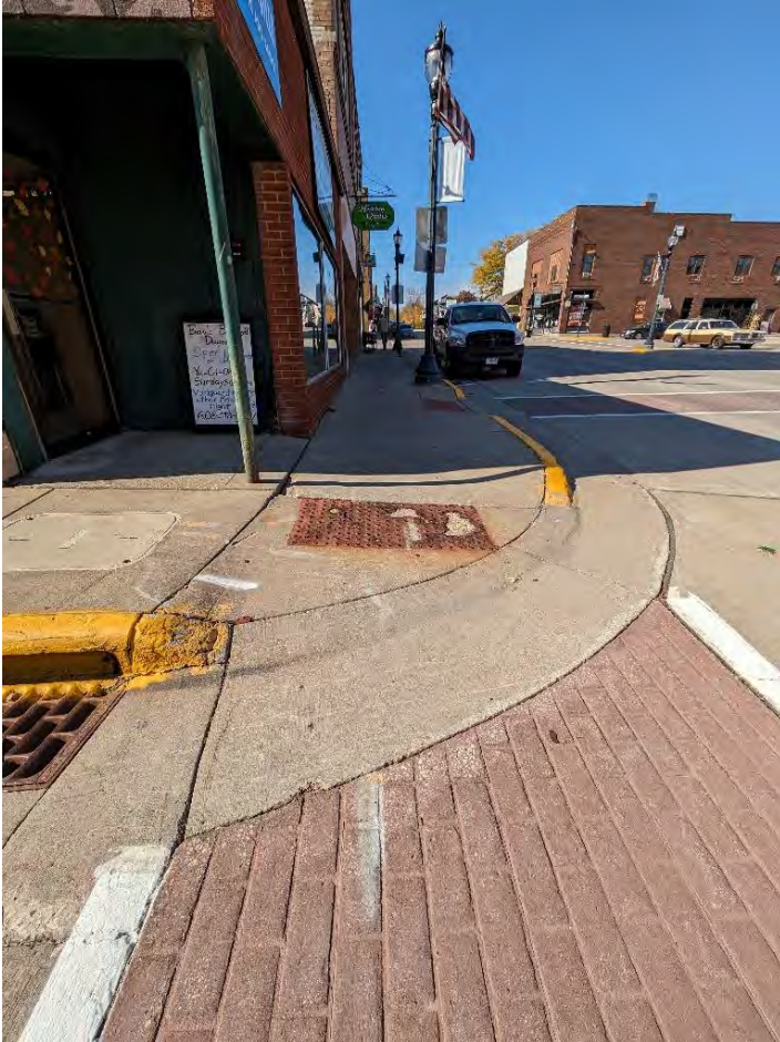
Figure 25: Broken ADA ramp (left, SW corner of Main and Bonson) and noncompliant ramp (right, SW corner of Southwest and Hickory)
