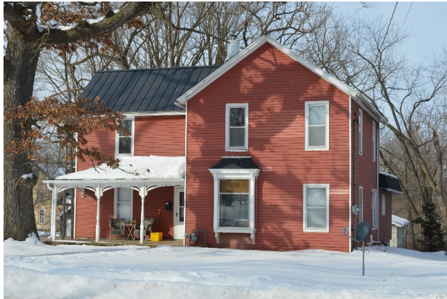
460 N. Elm St., AHI 46084, east elevation facing west.
