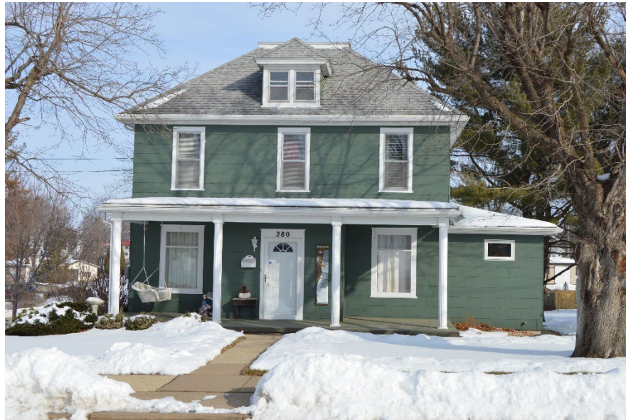
280 W. Lewis St., AHI 245436, south elevation facing north.
