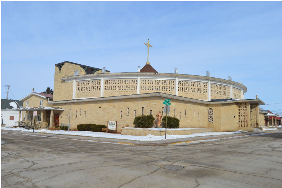
St. Mary's Catholic Church, 130 W. Cedar St., AHI 45884, east and north elevations facing southwest (top) and east and south elevations facing northwest (bottom).
