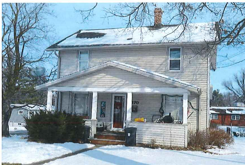
170 W. Lewis St., AHI 46155, south elevation facing north.
