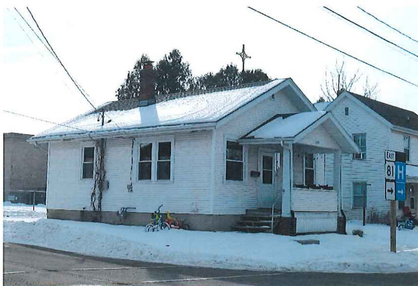
395 N. Chestnut St., AHI 45904, south and west elevations facing northeast.
