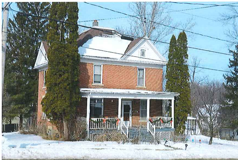
500 N. Elm St., AHI 46092, east elevation facing west.
