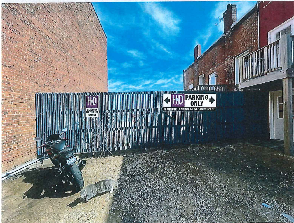
Mount using 2.5 " Pole Barn Screws into wood fence rails - Pre-drill first
