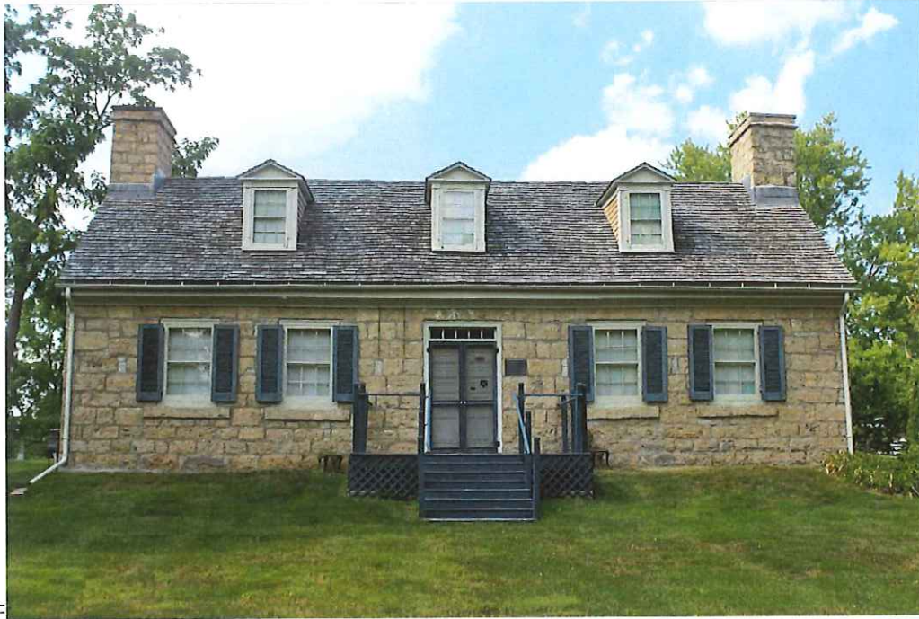
Front view (South facing)
