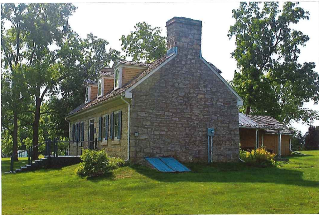
Side view, (East, southeast facing)
