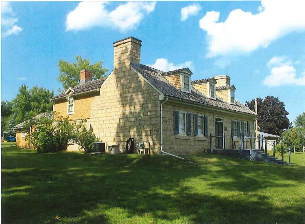
West, southwest view
