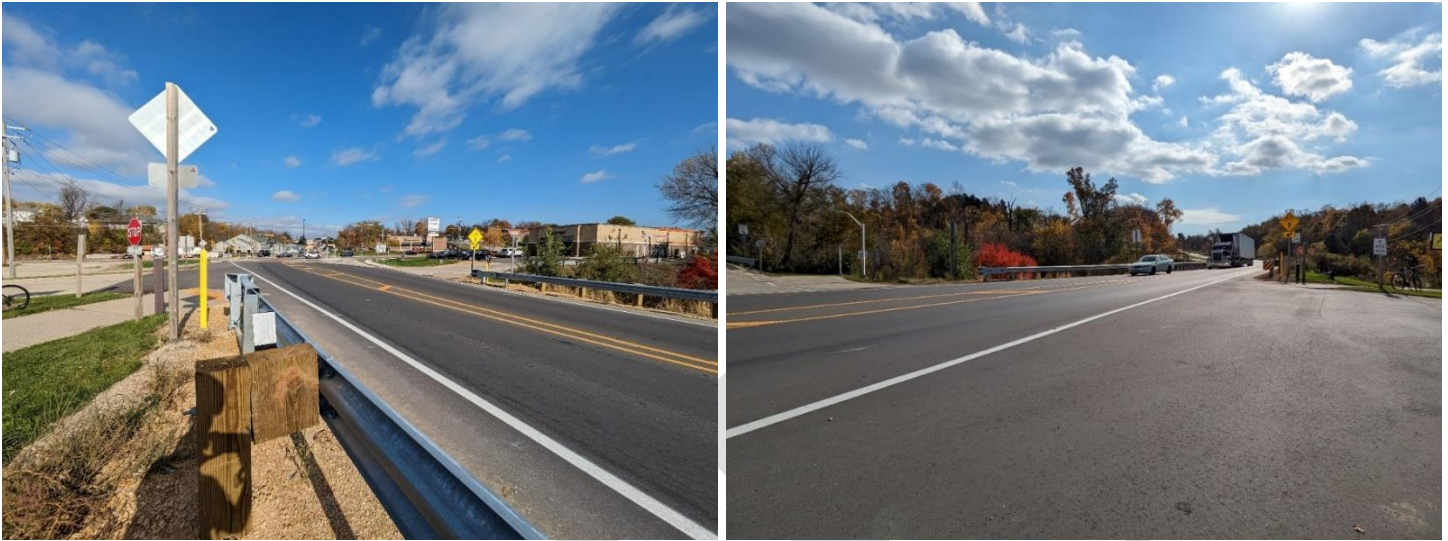
Figure 15: Northbound view of trail crossing (left) and southbound view with traffic (right)
