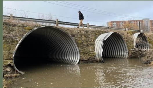
Figure 3: Existing Masonry Wall, Looking Northeast
