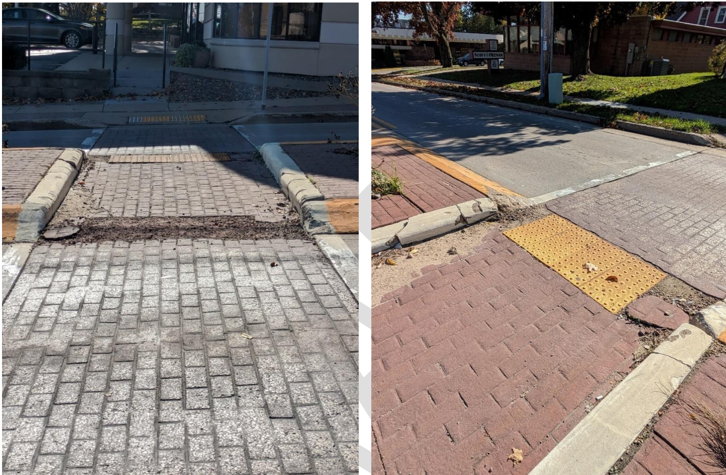
Figure 25: Pedestrian islands along Pine Street
