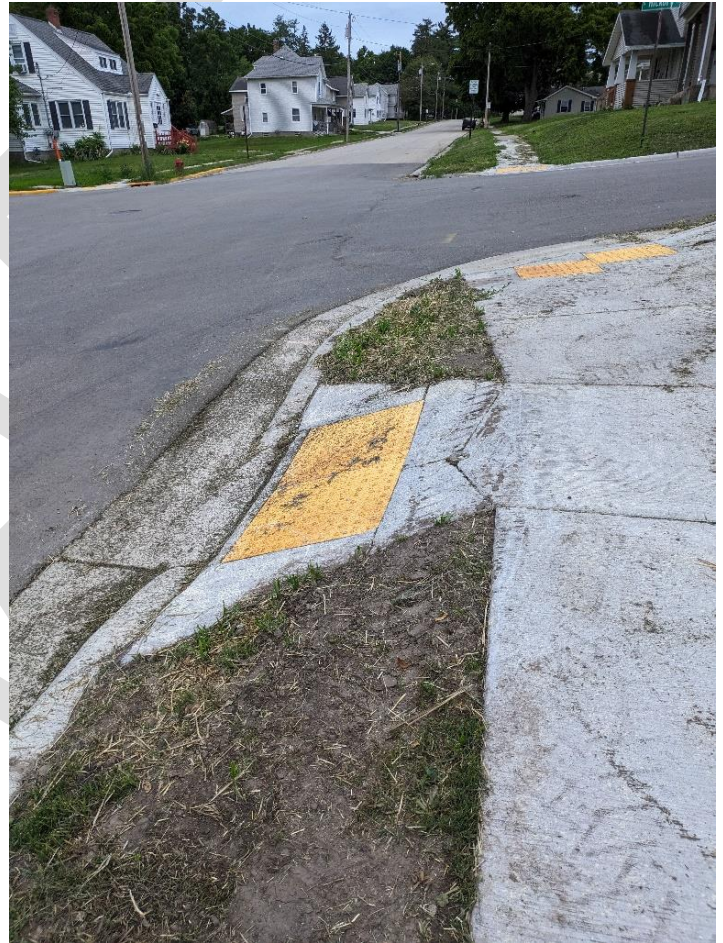
Figure 24: Broken ADA ramp (left, SW corner of Main and Bonson) and noncompliant ramp (right, SW corner of Southwest and Hickory)
