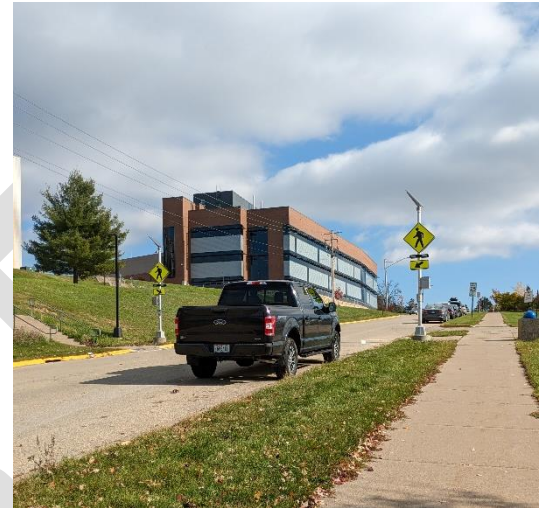
Figure 3: RRFB at Southwest Road and UWP Lot 28
