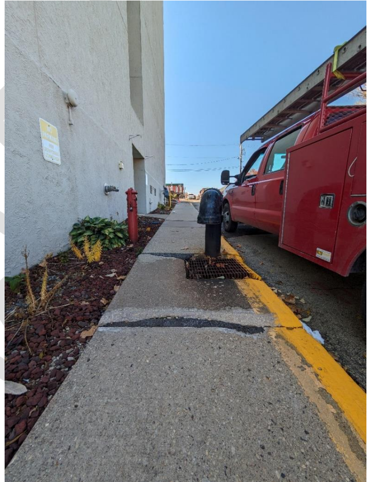
Figure 18: Cracks and uneven sidewalk on the south side of Mineral Street near Jenor Towers
