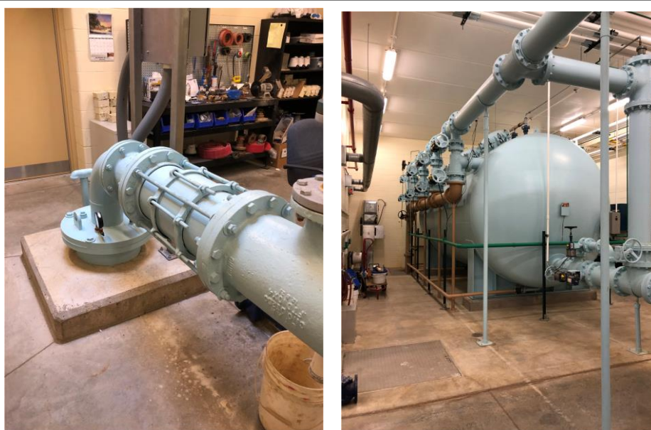
Figure 2.02-3 Well No. 5 Well Head and Filter System
