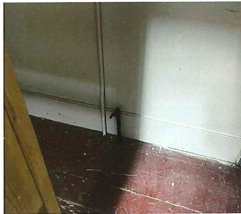
Figure 5: Remove gas line
