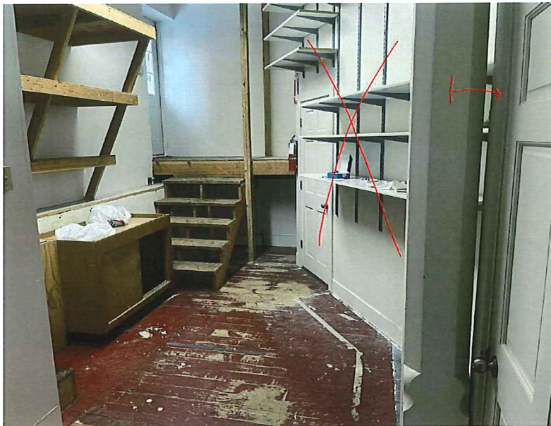
Figure 7: Waiting room. Support will shift 1ft to be within wall and steps redone
