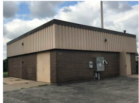
Figure 2.02-4 Well No. 6 Building
