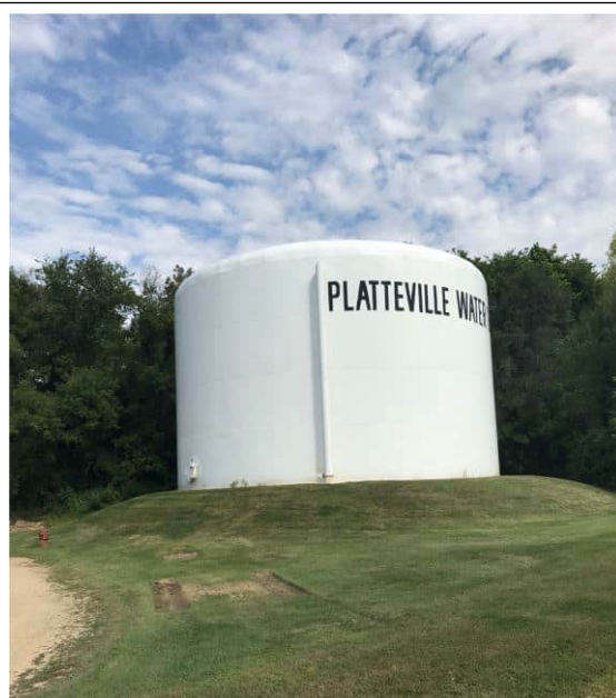
Figure 2.04-1 Davison Plant Reservoir
