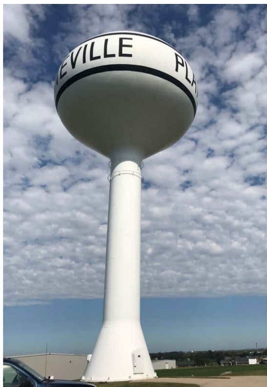
Figure 2.04-2 High Zone Elevated Tank
