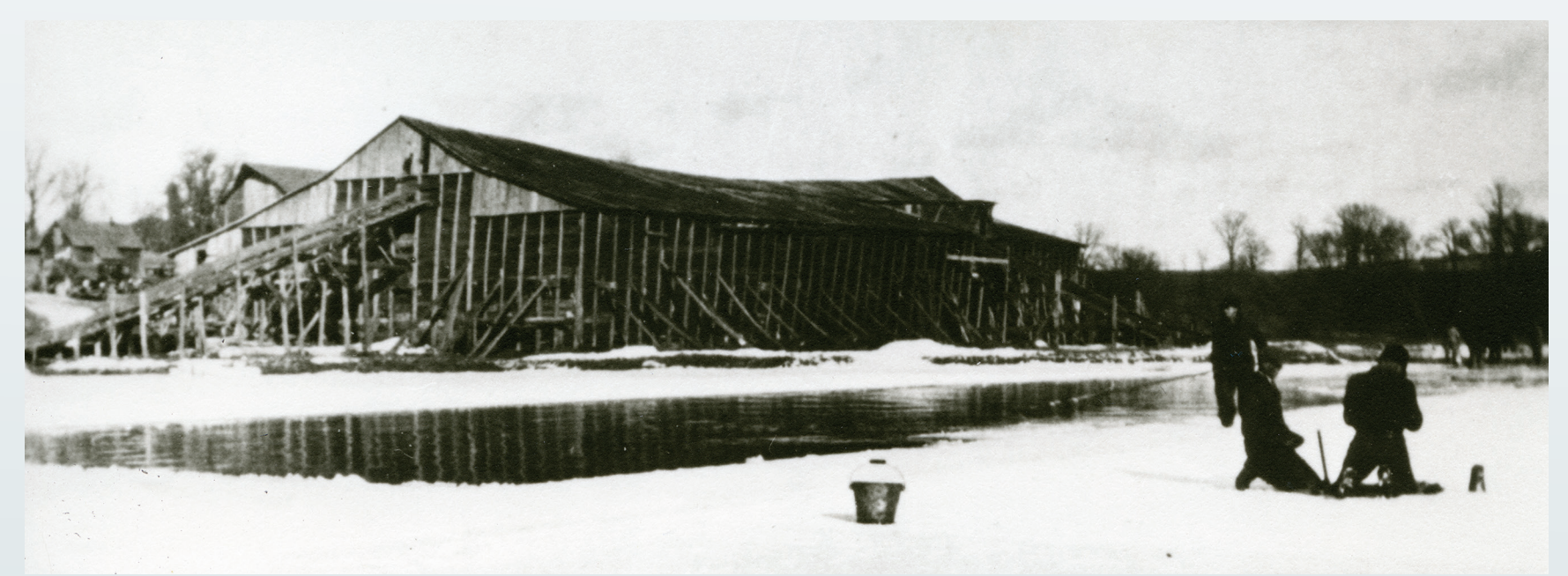
The largest ice house on this site was 120x 60 feet and 20 feet tall. It stood about where Culvers is now.
